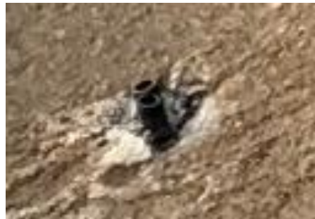
Photo 16B: Closeup of the existing tub for the piezometers
