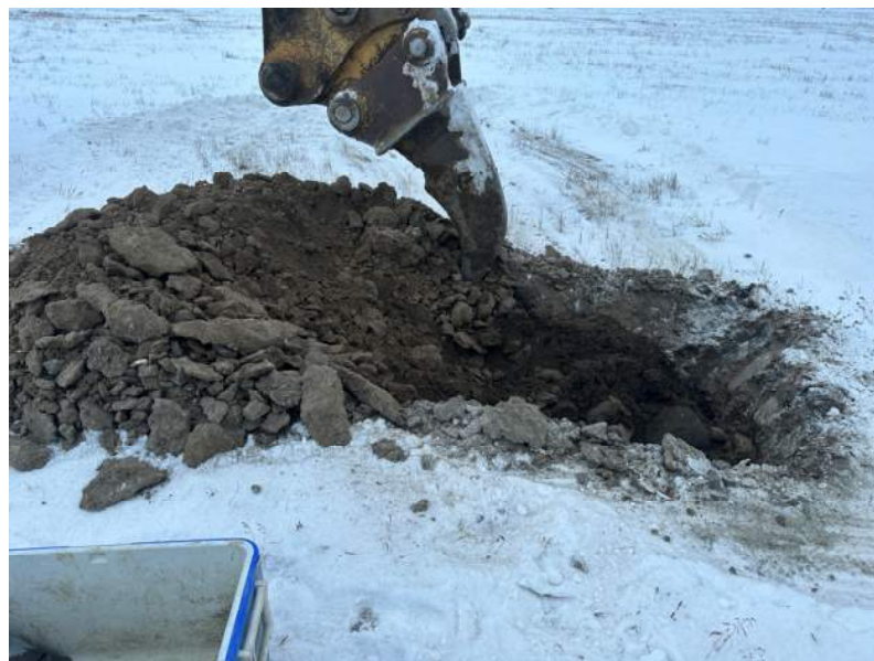
Photograph 10 Ripping frozen surface at TP18.
