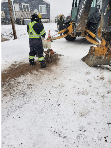
Photograph 1 – September 21, 2021 Cutting through asphalt for TP01.
