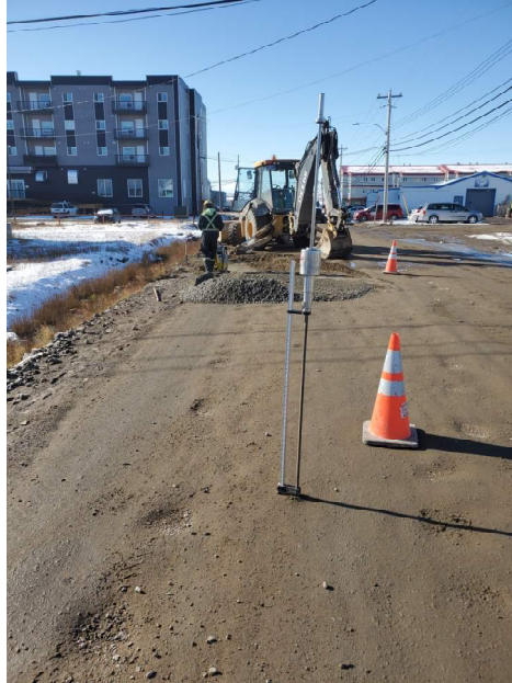
Photograph 11 – September 23, 2021 Dynamic cone penetration testing adjacent to TP07.
