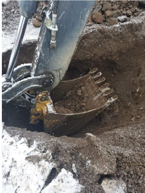
Photograph 5 – September 22, 2021 Excavating TP04.
