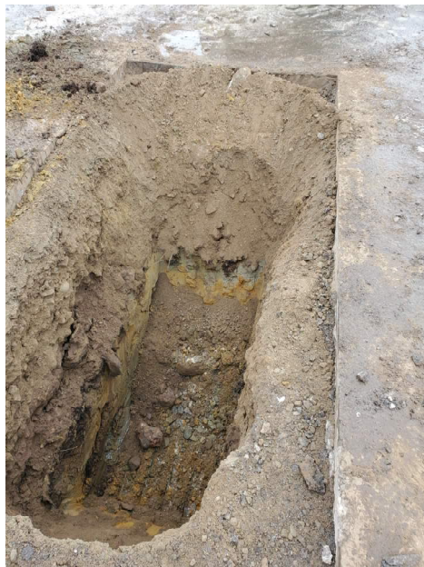
Photograph 2 – September 21, 2021 TP01 after excavation.
