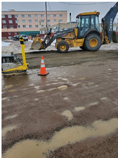
Photograph 8 – September 22, 2021 Grading backfill surface of TP05.
