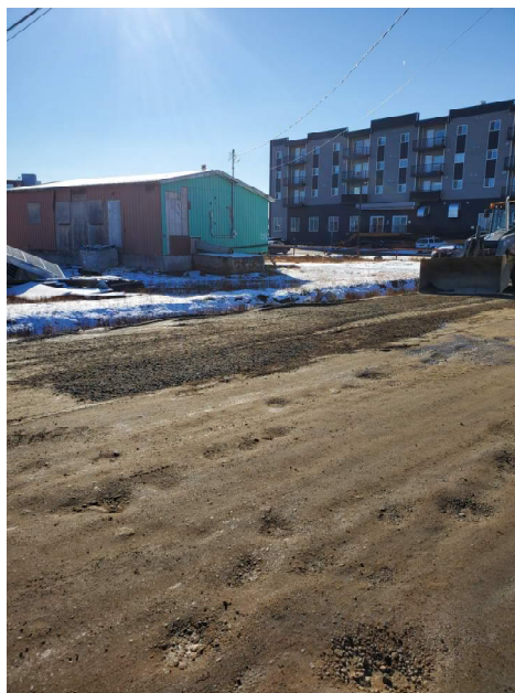
Photograph 12 – September 23, 2021 Location of TP07 after completion of work.
